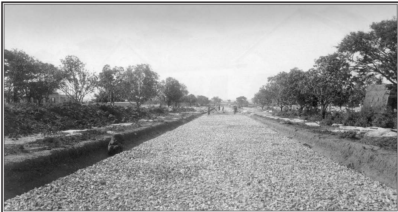
Alluring Gulmohar Marg to ECE Department (While under Construction)
