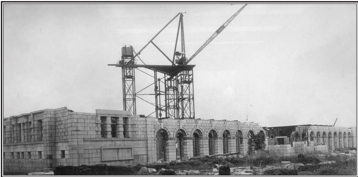
Main Building Under Construction
